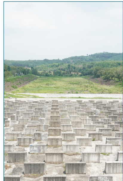
c. Ground seal at Jatiluhur spillway
